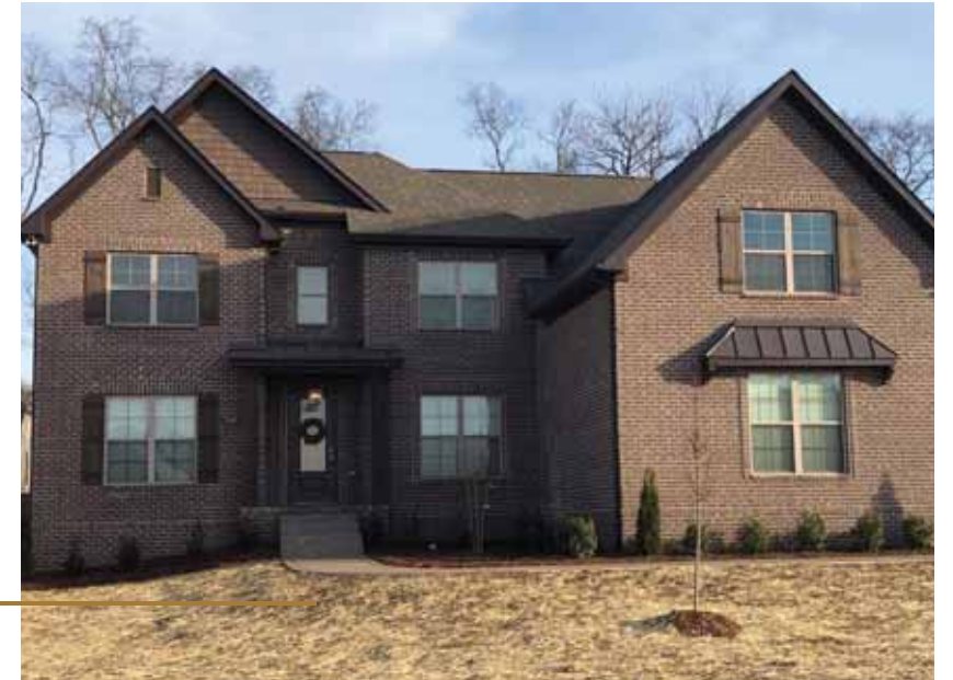
Shiloh Falls Brown Upgrade Mortar
