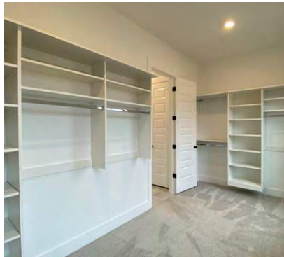
Closet with Melamine Shelving
